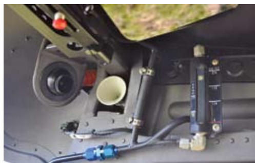
Not hiding the plumbing behind cabin trim at least allows easy inspection of components, and the fuel sight gauges are the simplest and most accurate possible. The stall warning horn is — a horn.
